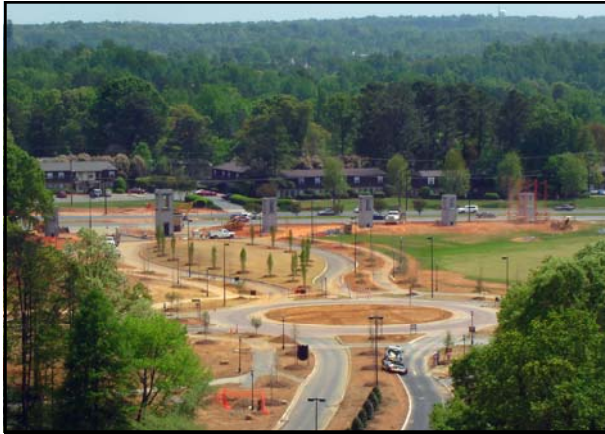
New Front Entrance - Photo taken by Wade Bruton, University Photographer
